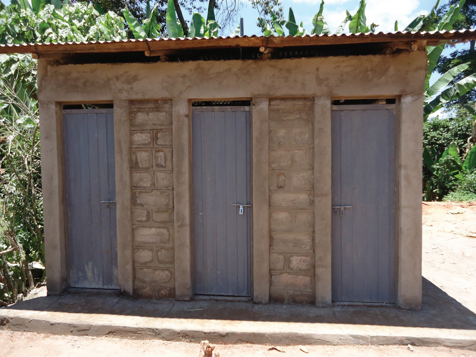
Latrines Constructed in Bule Hora Woreda (2015)
