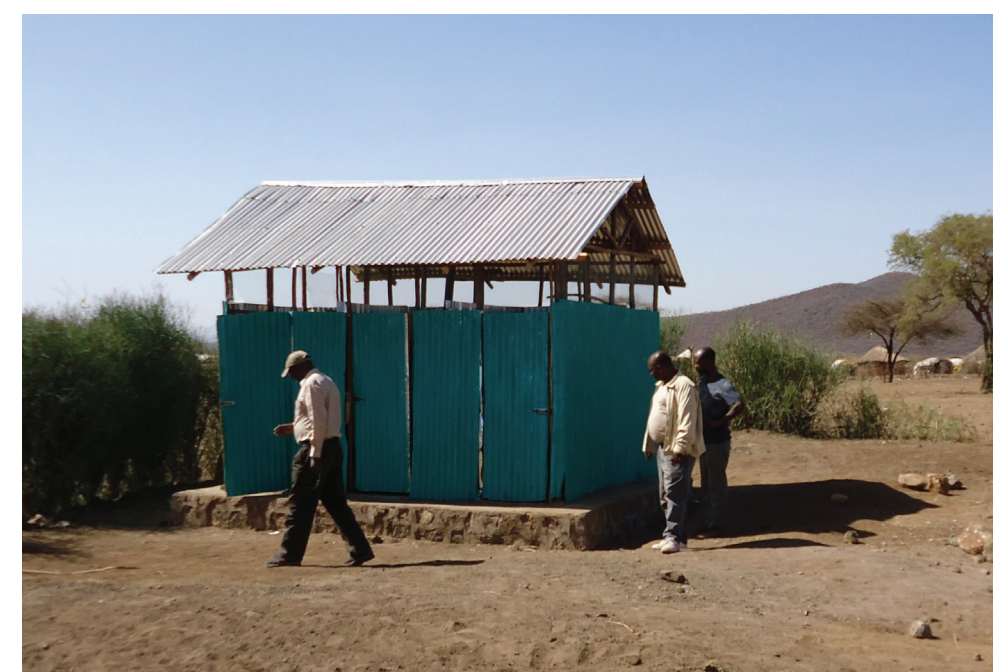
Latrine Finishing Works Completed in Ngunyyiel Refugee Camp, Gambella
